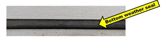
If it isn't OK, replace it and recalibrate the door opener if any before installing the RodeXit seal. Take care to observe all security instructions in the owner's manual.
