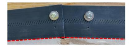
Two pieces installed by means of crews and washers overlapping and at an angle
