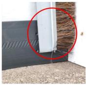
Tucked under brush side seal installed on the door.
