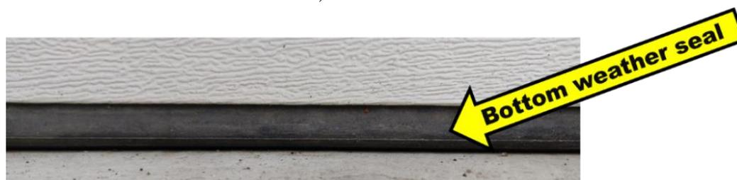
If it isn't OK, replace it and recalibrate the door opener if any before installing the RodeXit seal. Take care to observe all security instructions in the owner's manual.
