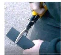
10) If there is a right side seal, tuck the free right end of the trimmed seal behind the side seal:
